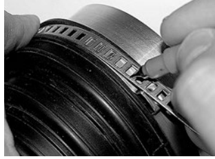
Step 2 Determine the clamp length.
